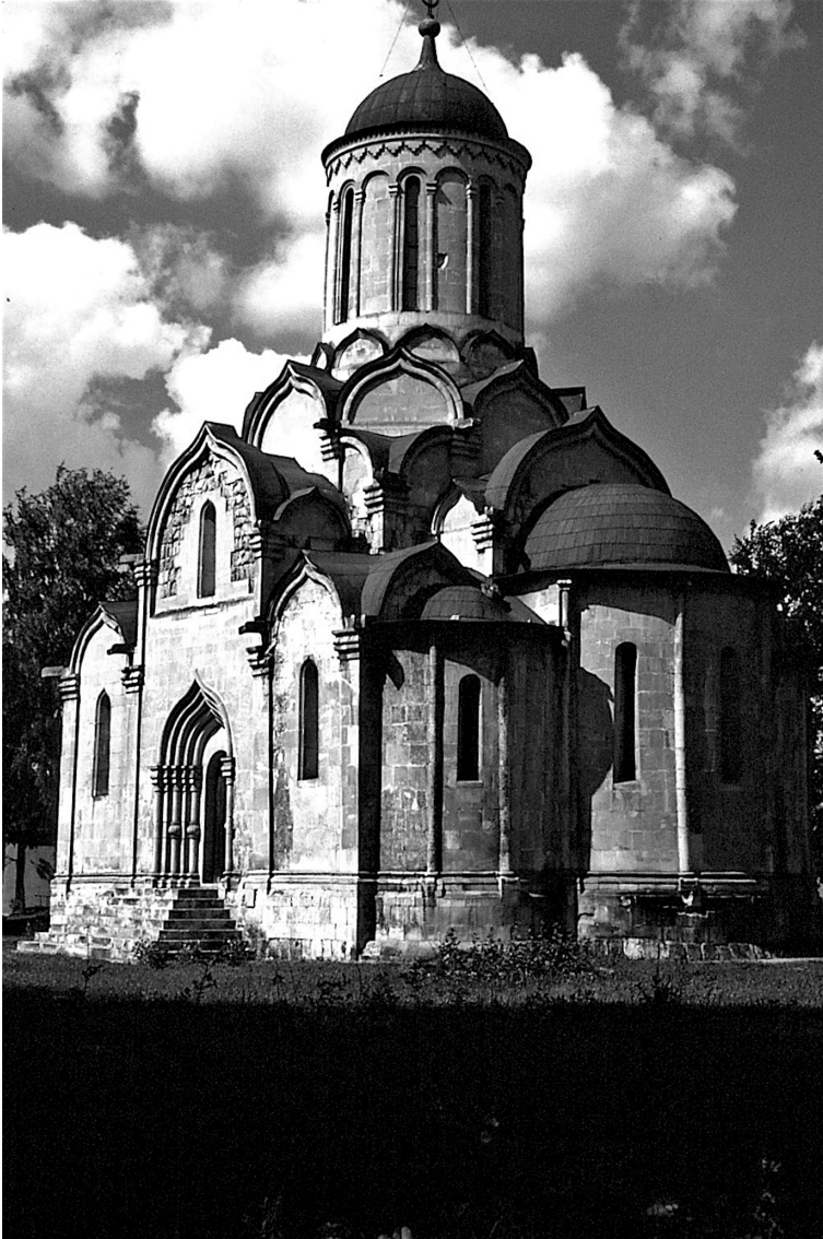
FIGURE 24.3. Andronikov Monastery, church, Moscow, 1425–1427, exterior from southeast. Photo: Mark J. Johnson.
